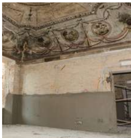
05 Make a first float finishing.
