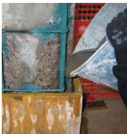
05 Pouring of the ADEGROUT FLUIDO grout in the form.
