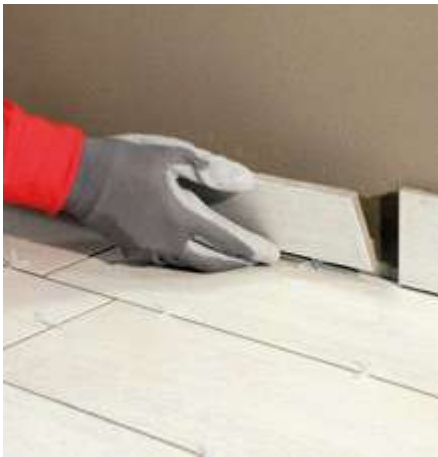
07 Install the skirting boards.
