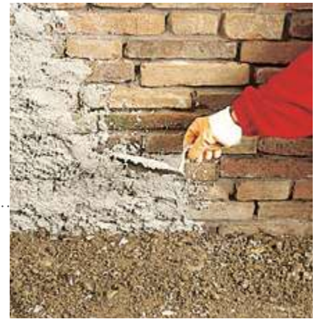
03 Apply an even coat of ADESAN RINZAFFO CALCE.
