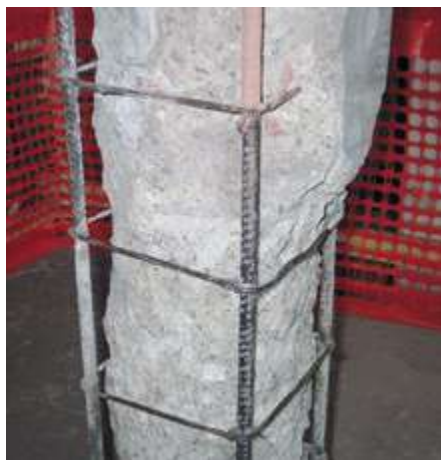
01 Removal of deteriorated parts.
