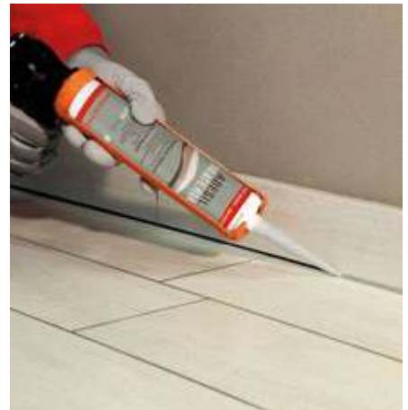
09 Seal the floor to wall joint carefully with the silicone sealant ADESIL MATERIA .
