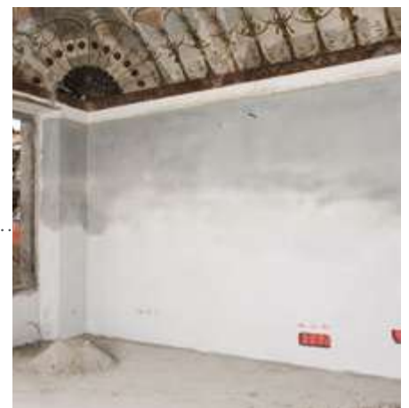
06 Level with ADESAN RASANTE (fine white coat finishing).
