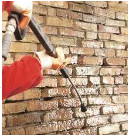
02 Carefully wash with pressure water.
