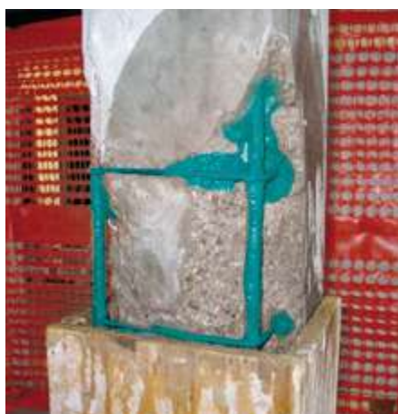
04 Form positioning and substrate wetting.
