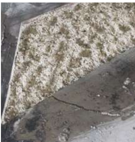
04 Saturation of the substrate with water, and possible removal of stagnating excess water.
